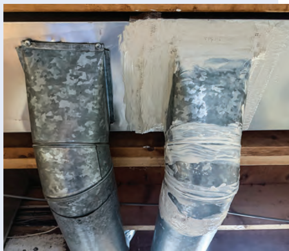
SEAL IT UP A side-by-side comparison shows where to apply mesh tape and mastic to close gaps around metal ducts.
